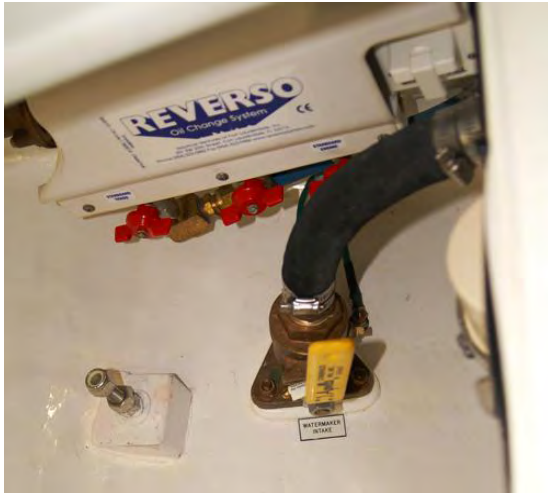
Turn through hull valves and service if needed
